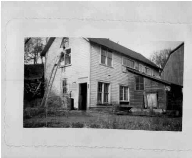
The ca.1926 milk plant being refurbished in 1948
