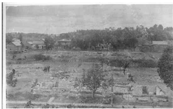
In the foreground is Maple Ave. showing the cellars of the destroyed houses. Looking across the central area to Factory St. can be seen the Grieve house, then the square house where John Stoffel now lives and the house where Greg Brown lives. At far right is the cheese factory. These pictures can be seen as a panoramic view, mounted on a cardboard backing, in the Edwards History Center.
