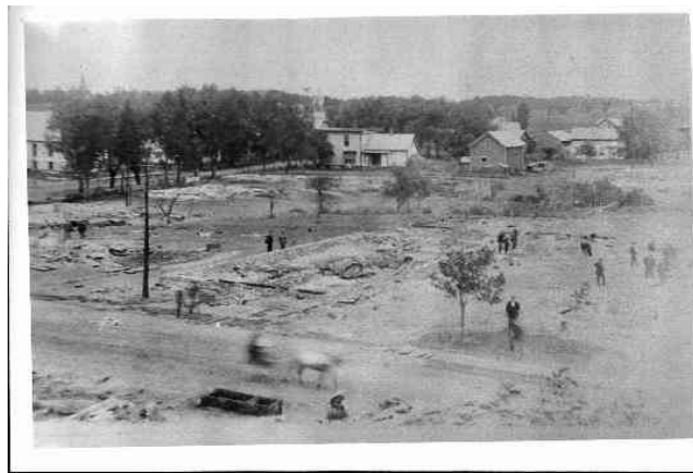
Overview of area between Maple Ave. and what was then, Factory St. (now Court St.). Shows Alvin Gardner's house, which was spared. The fire burned Dr. Taylor's just before Gardner's, then changed directions going to Factory St. burning the buildings on one side of the street. In the background can be seen one of the oldest houses in the village, occupied at that time by Mrs. Grieve and someone else. At that time it was a double house. Now it is painted blue and occupied by only one family.
